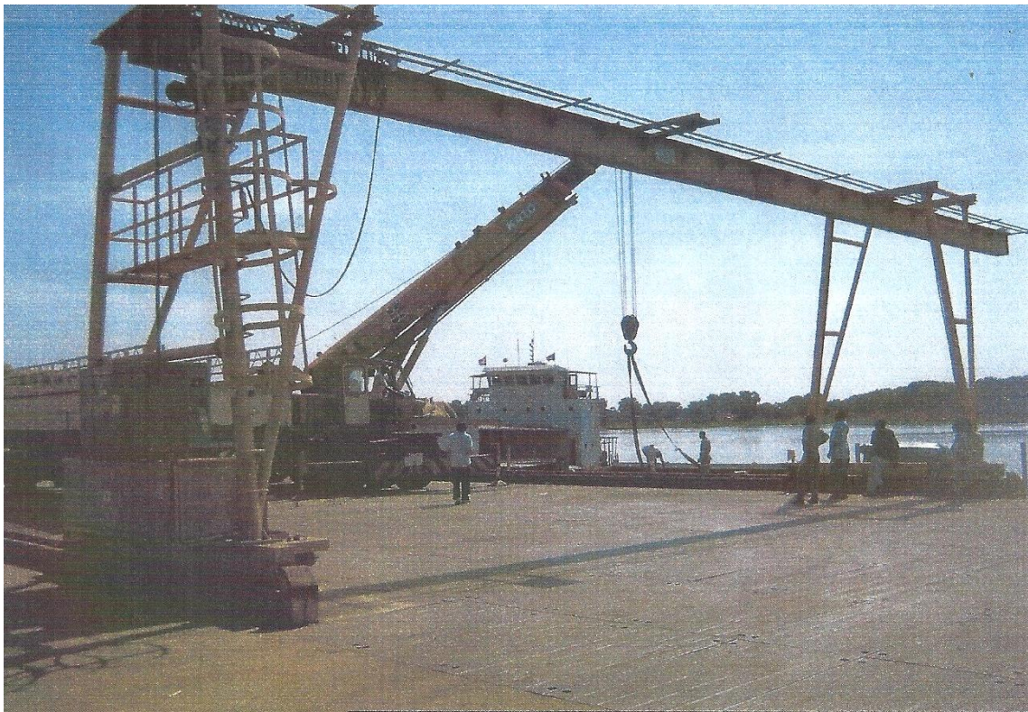
Fig.2. Gantry crane on Juba River Port (Donated by Japan in 2007)
